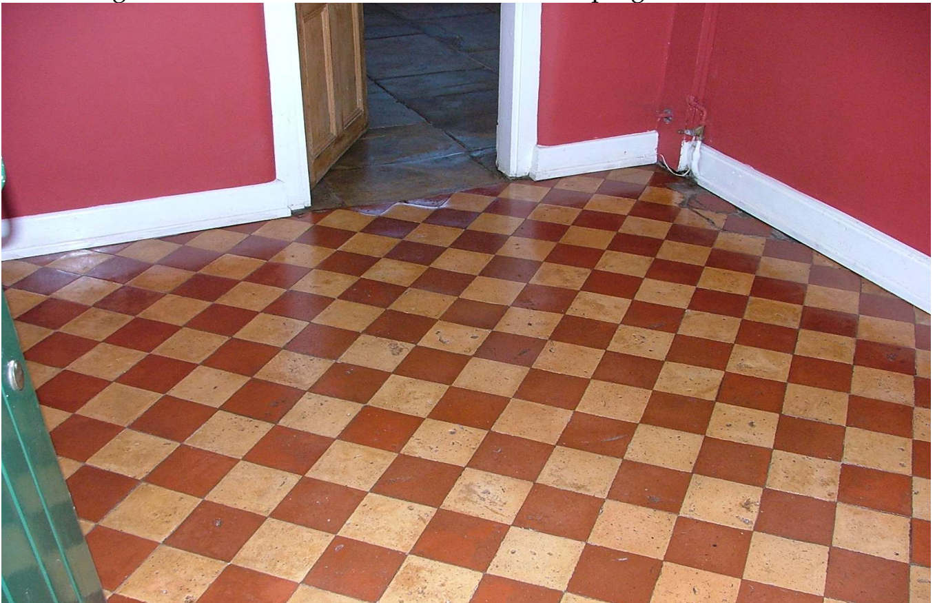
Victorian geometric tiles restored cleaned & sealed.
