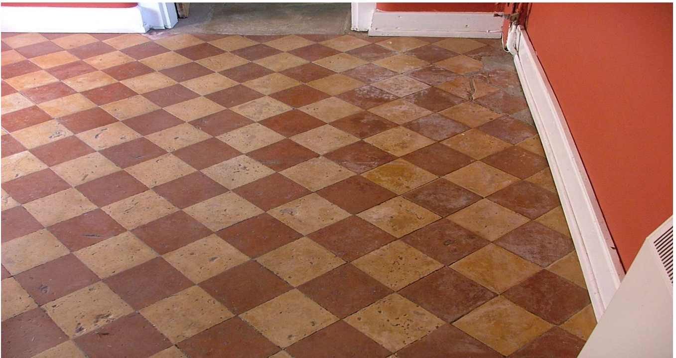
Victorian geometric tiled floor before restoration. Top right shows efflorescence.
