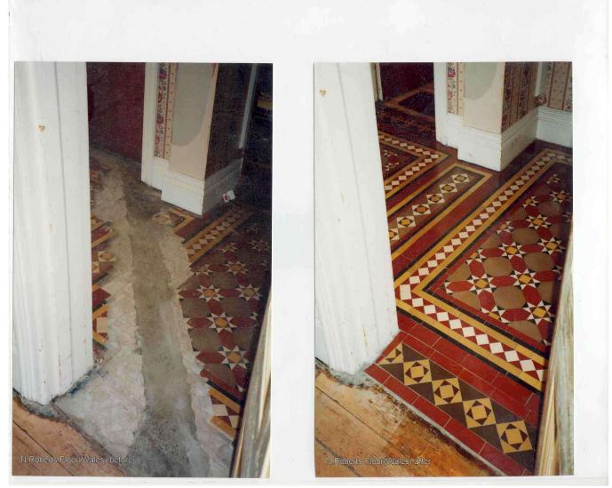
This floor was restored before the advent of Exakt saws & Fein SuperCut. To preserve the edges of the firm unbroken tiles I took out the concrete infill from the middle working towards the tiles carefully, but as was usual working in this manner many of the tiles surrounding the infill worked loose due to the percussive effect of the hammering using cold chisels.
