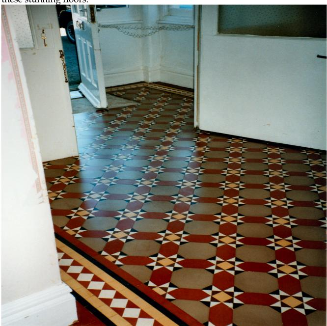
Stunning floor in Llandudno picture shows the matwell. A section of tiles were lifted to make a matwell as this would keep the floor looking its best if muck etc was removed first. P3.
